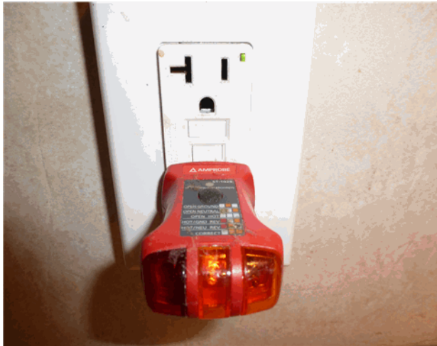
Open ground on GFIC
