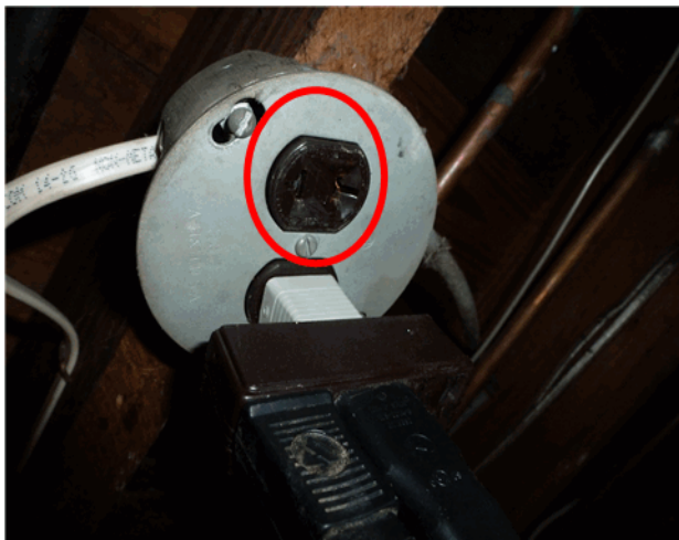
Electrical outlet above cloths washer has no ground.
